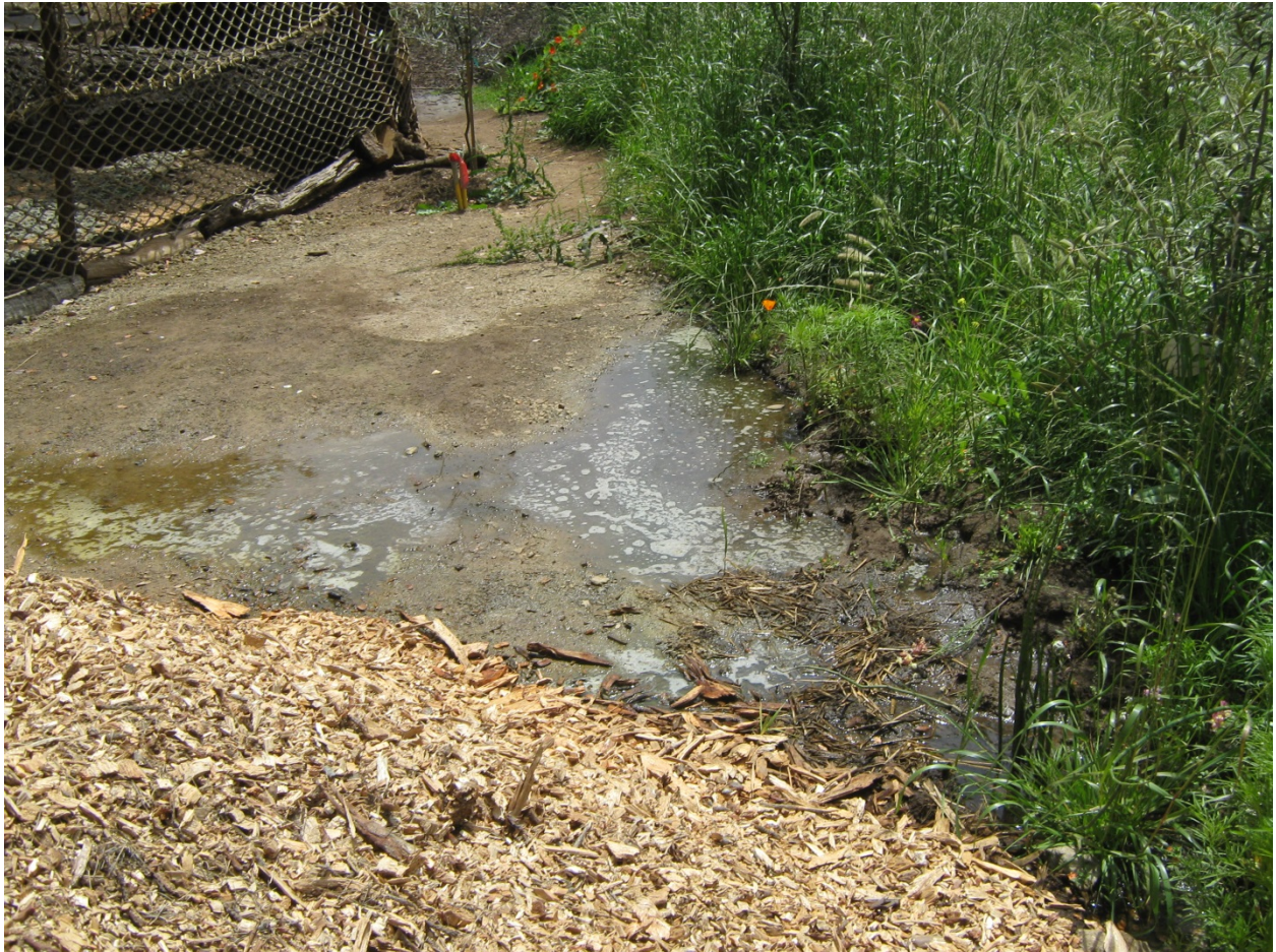
Surfacing Effluent North End of Drain Field
